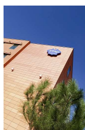
Etap Hotel Toulouse Airport
