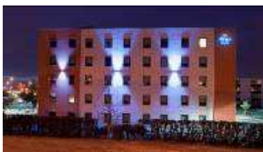
Etap Hotel Toulouse Airport, Francia
